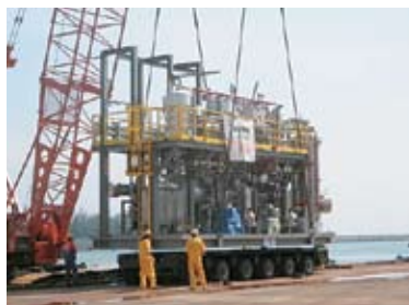
Skid loaded on Barge
